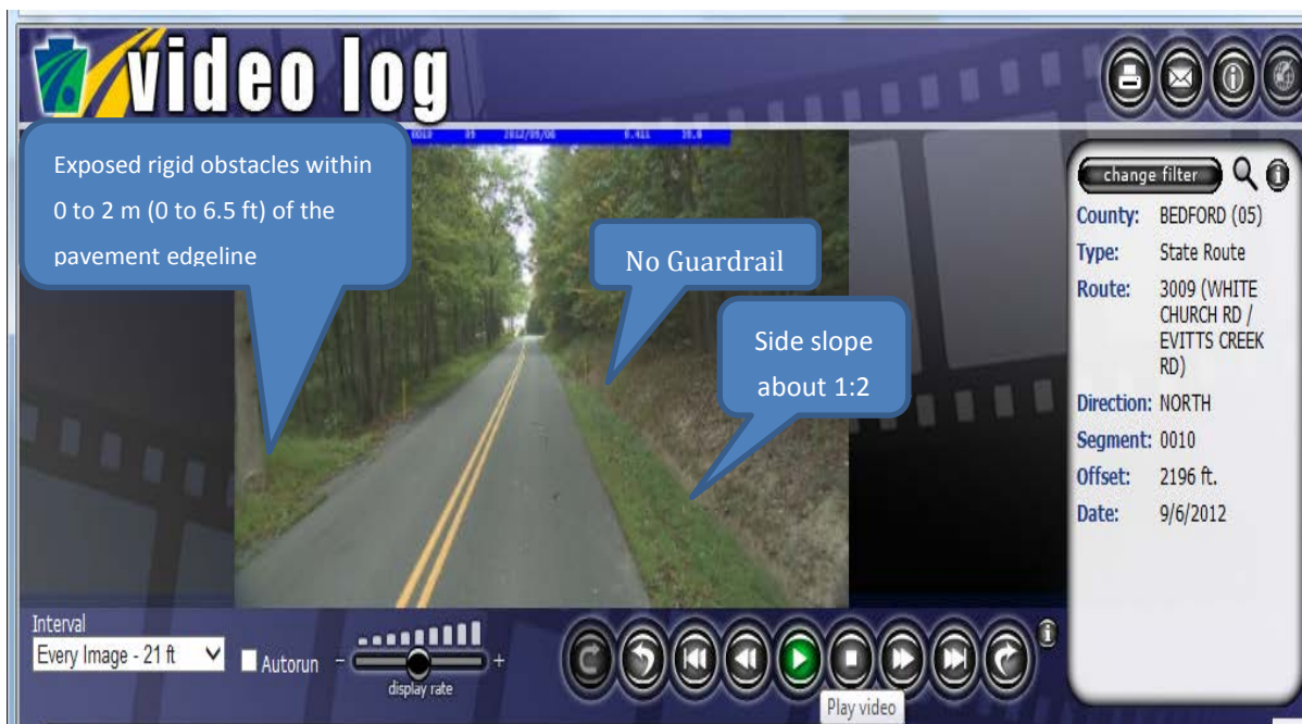
Figure A17. Video Log for SR 3009 Segment 0010.
