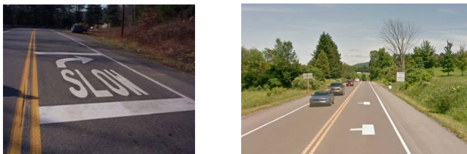
Figure A24. Example of horizontal curve warning pavement marking (left panel) and intersection warning pavement marking (right panel).
