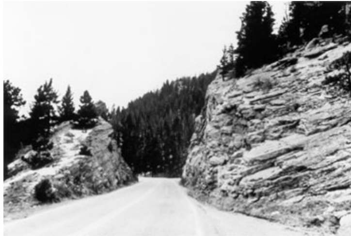
Figure A15. Roadway with Roadside Hazard Rating Equal to 7.
