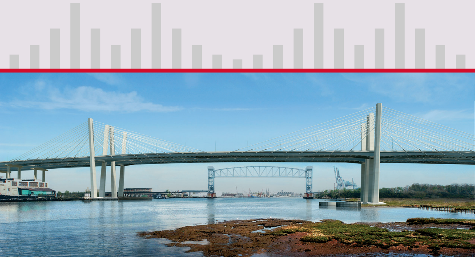
Goethals Bridge Replacement, New York & New Jersey Macquarie
