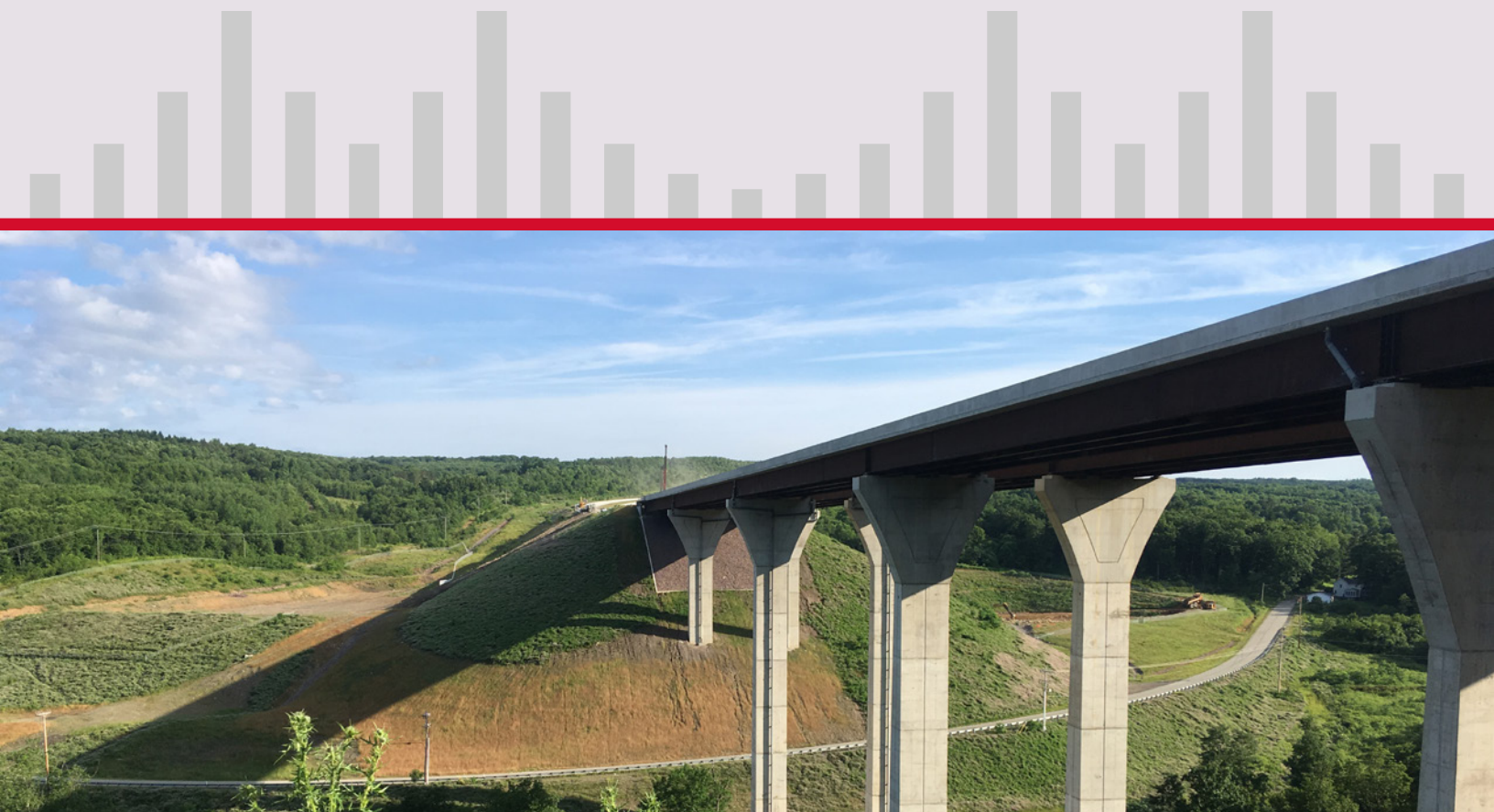
US 219 New Highway Construction, Pennsylvania Fay
