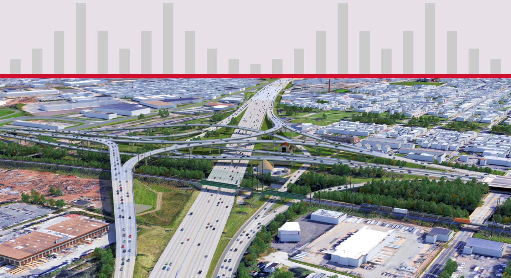
I-95 Section BRI Reconstruction, Pennsylvania STV
