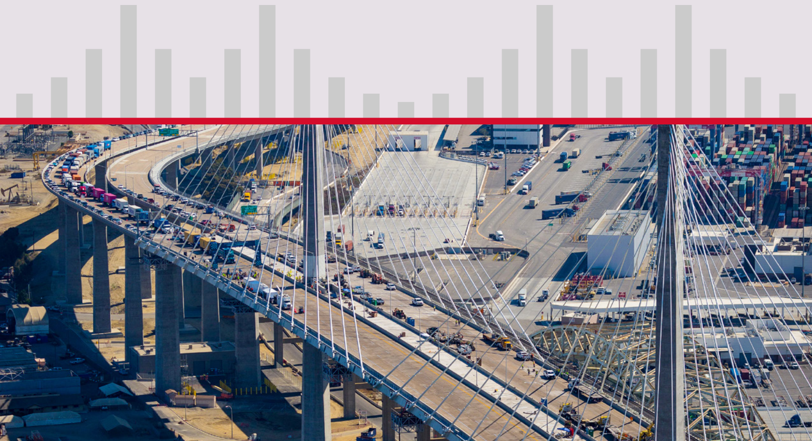
Gerald Desmond Bridge, California FCC
