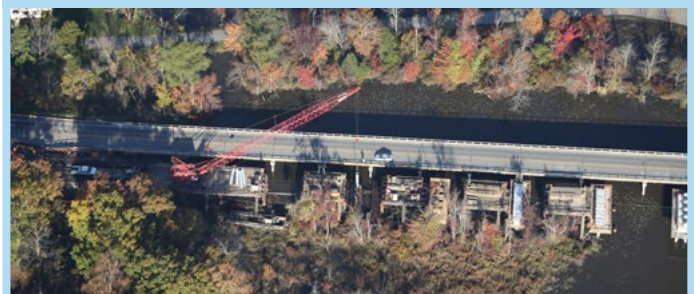
FIGURE 3 - TUCKAHOE BRIDGE TEMPORARY TRESTLE
