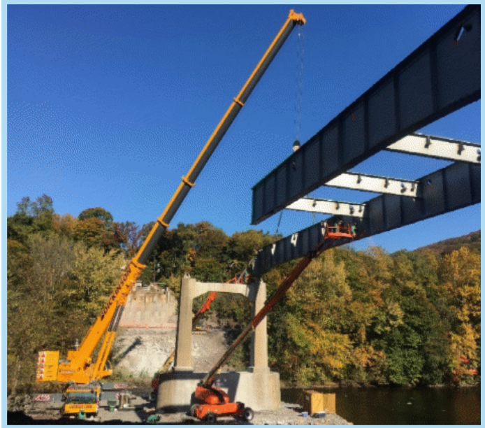
FIGURE 10 - STEEL REMOVAL AT JIM THORPE BRIDGE
