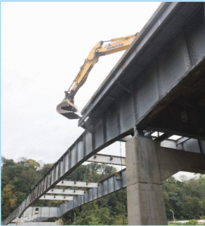
FIGURE 9 - DECK LIFTING AT JIM THORPE BRIDGE
