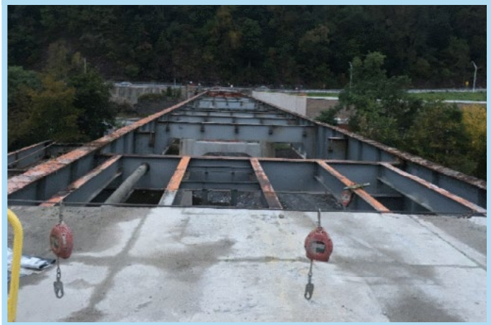
FIGURE 8 - DECK AND SELECT STEEL REMOVAL AT JIM THORPE BRIDGE
