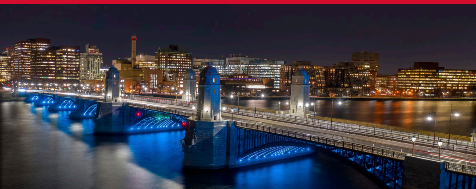
Longfellow Bridge Rehabilitation, Massachusetts STV
