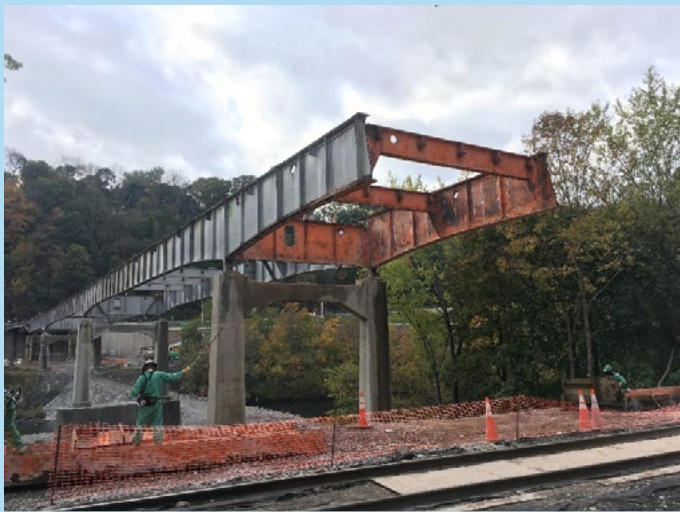
FIGURE 12 - STEEL REMOVAL AT JIM THORPE BRIDGE
