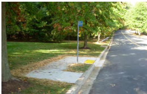
Image of a curb height ADA loading pad for bus stop in Montgomery County, MD
