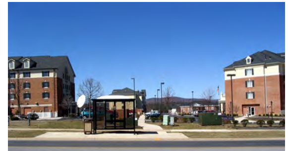
Bus stop infrastructure and pedestrian connections implemented as part of the land development process due to coordination with CATA.
