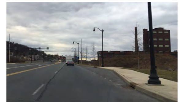
Bus bays along Fourth Street (SR 412) in Bethlehem, Northampton County
