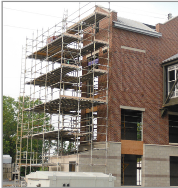
Middletown Train Station
