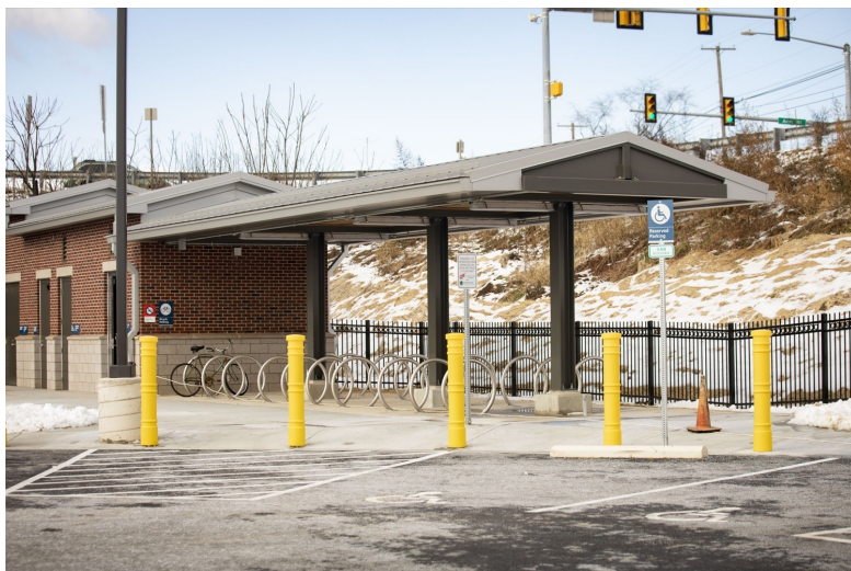
New Middletown Train Station
