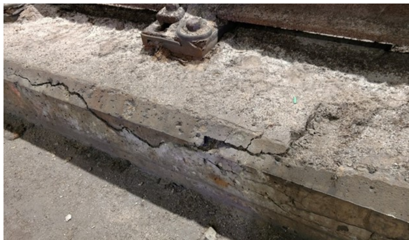
Top: New LED tunnel lighting in the CBD Tunnel Bottom: Degrading concrete plinth to be rehabilitated in CBD Tunnel
