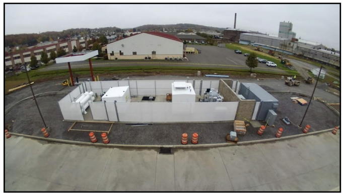
BTA-Butler CNG Compressor Compound under Construction.
