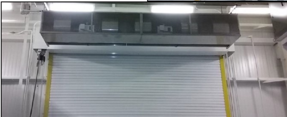
Various facility improvements included in the BTA CNG Facility Modifications and Upgrades project
