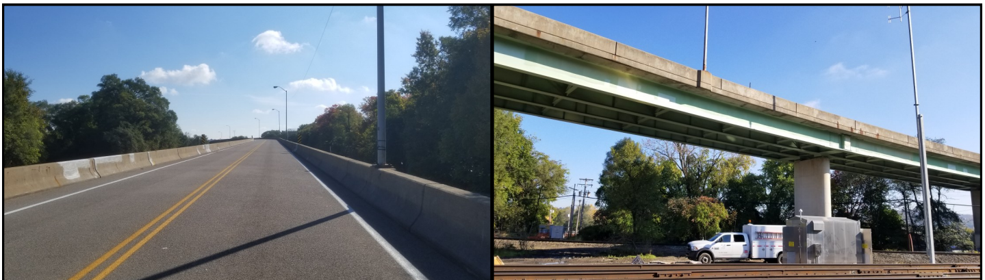
Brilliant Viaduct Bridge before and after rehabilitation
