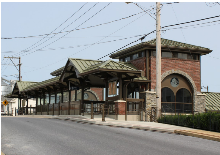
Left: Mount Joy Station, completed in 2019 Right: Paoli Station, completed 2019
