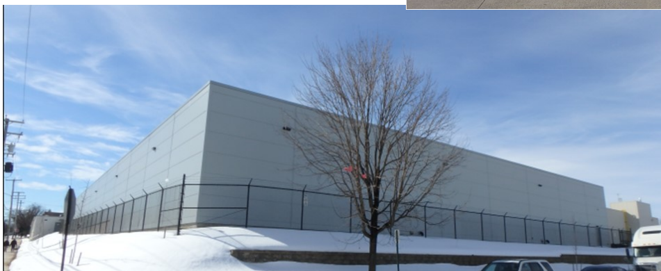
SCTA bus garage after construction
