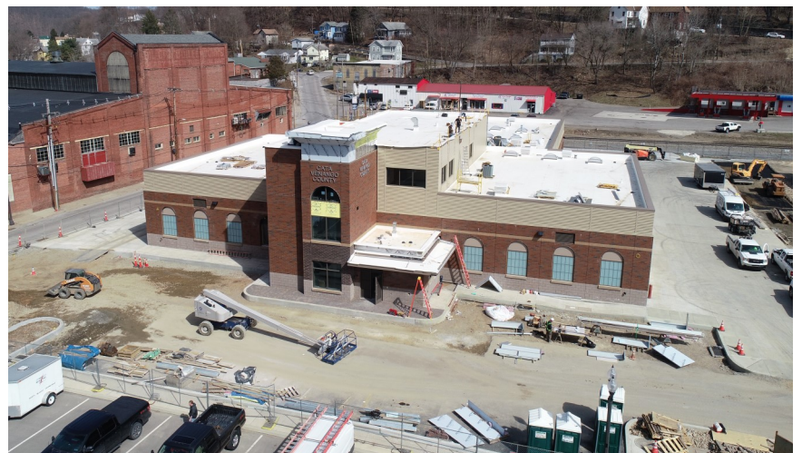
CATA Oil City Operations and Maintenance Facility
